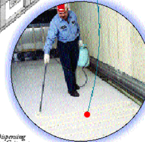
► Dispensing Insta-Grip onto fiberglass liner
