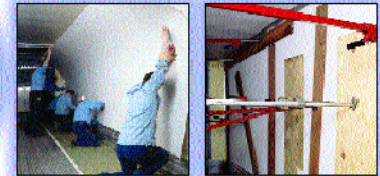
► Liner placed onto trailer wall. Bracing installed to maximize bonding process
